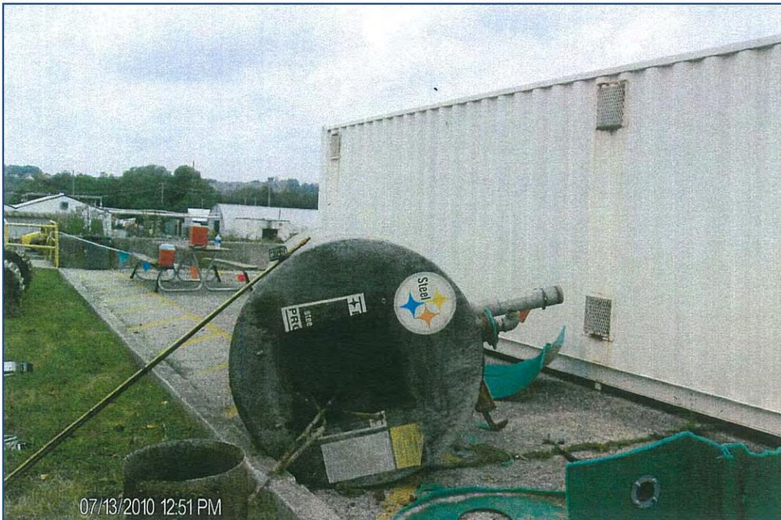
**Tank 010 (1,000-gallon diesel fuel) following removal.**
