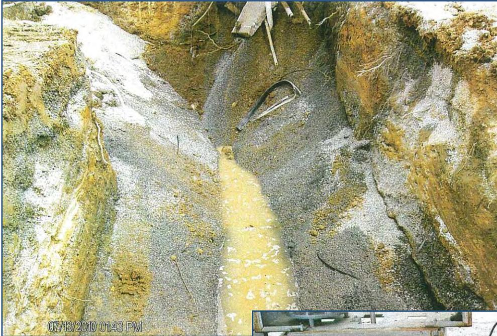
**Tank 009 (10,000-gallon unleaded gasoline) excavation following removal of the UST. Note water at the base of the UST excavation.**
